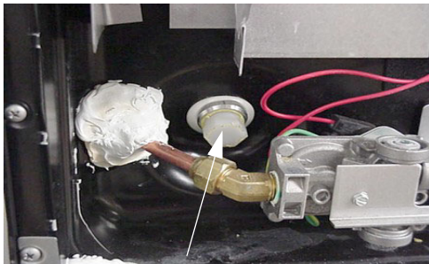
Water Heater Drain Plug (Remove with socket)
